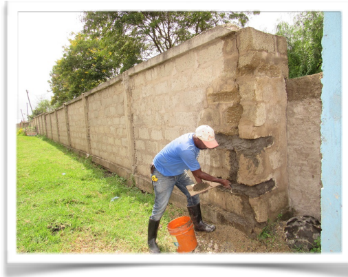
Repairs to the orphanage wall
