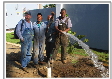
Water drilling team with a new well
